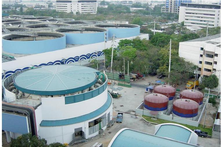
Privately operated by Utility Business Alliances Co. Ltd., the Dindaeng facility has a treatment capacity of 350,000 m<sup>3</sup> per day. All seven plants combined can treat only 40% of wastewater generated due to limited plant capacity to handle both wastewater and storm water runoff. During the wet season the river's flow is twenty times that of the dry season, causing a vast seasonal fluctuation in the pressure on the wastewater treatment system because of the stormwater flow.
